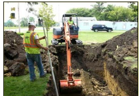
network. Large, deep trenches are rarely needed with pressure sewers. The shallower trench width and depth results in minimum surface disturbance, and quicker restoration. Directional boring can reduce highway closures and other urban disruptions and save both time and money. The small diameter piping is flexible and can be routed around obstacles. Pressure sewer mains can often be located on the shoulder of the road.
