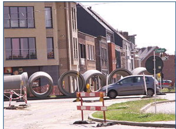
*Larger flows require larger diameter pipe for gravity sewer systems. Deeper (and more expensive) excavation is also needed but the cost may be offset by the fact that pumps and lift stations are only required in areas with inadequate slope for gravity flow.*
